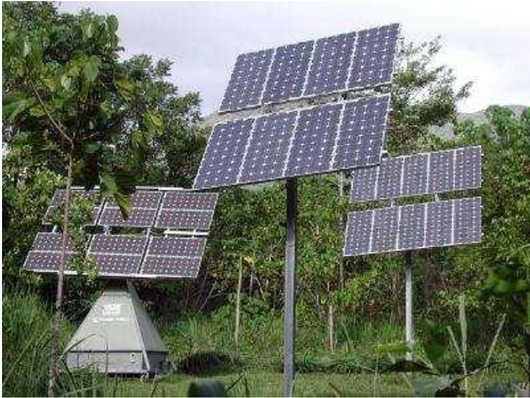
Appendix 2 Fig 3 Solar array at the Cape Tribulation Tropical Research Station. 30 BP 85 watt panels and two types of Suntron trackers. The original tracker is on top of the Pyramid Power packaged RAPS system supplied to the Station in 1995 (its alignment has drifted, as can be seen by comparison to the other two arrays.). Peak installed output 2550 watts. The front tracker was installed in Jan 03.
