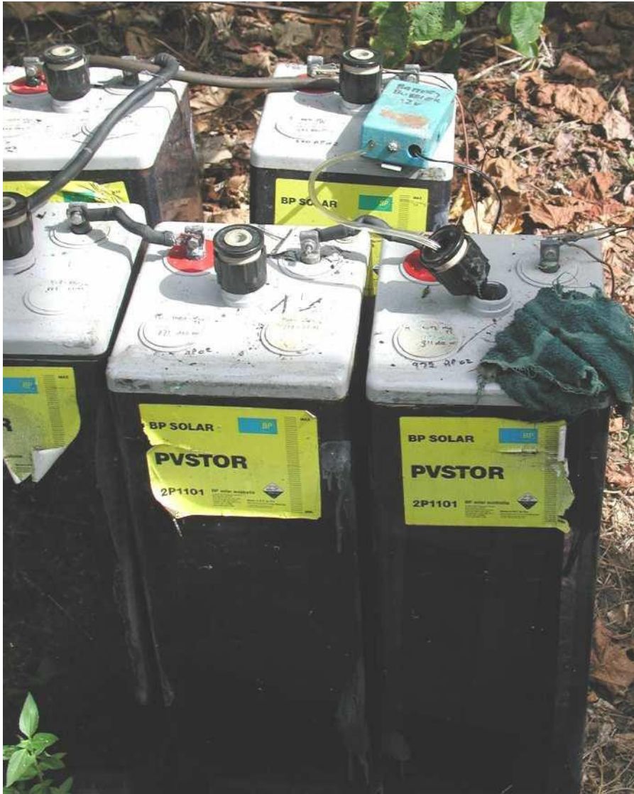
Figure2 A battery driven bubbler (small blue box) with its output tube inserted into the side of a PVStor cell. These cells have been removed from the system, but are still useable, and are being trickle charged from the main Array while being held as spares for other failing systems in the area.
